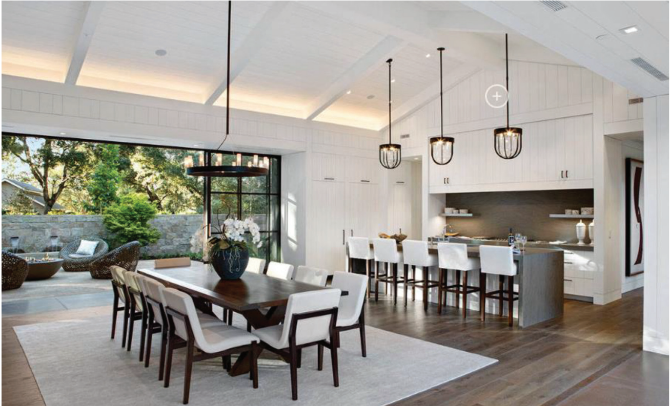
Concept Photo Vaulted Ceiling – Wood Beams Painted Trim Color W/ Lighting, No T&G
